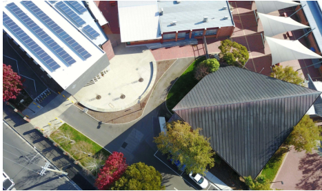
St Pat's Aerial View
