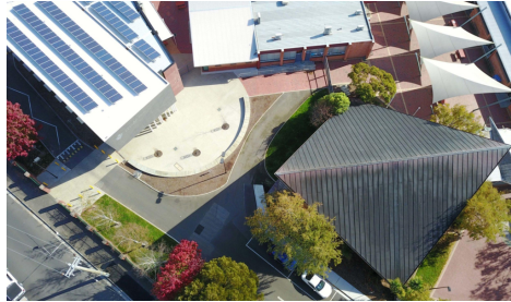
St Pat's Aerial View
