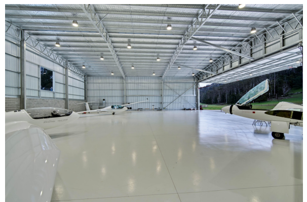
The VALE Aircraft Hangar 000021
