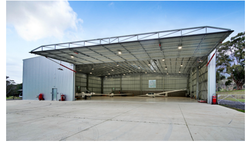
The VALE Aircraft Hangar 000111
