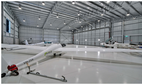
The VALE Aircraft Hangar 000141
