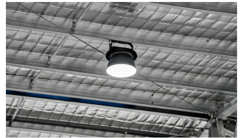
The VALE Aircraft Hangar 000231
