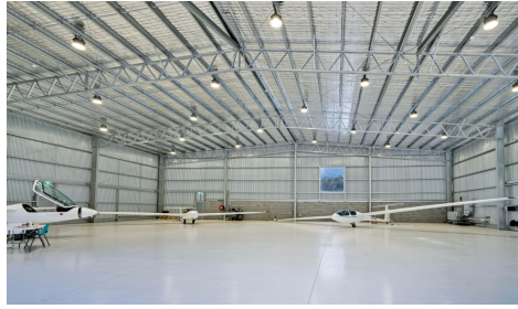
The VALE Aircraft Hangar 000091
