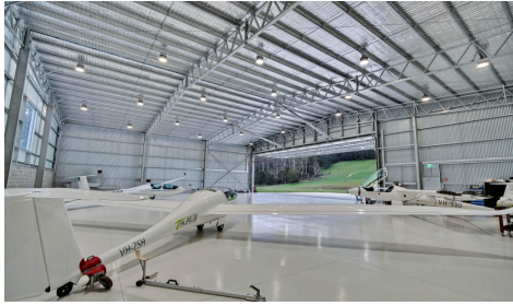
The VALE Aircraft Hangar 000041
