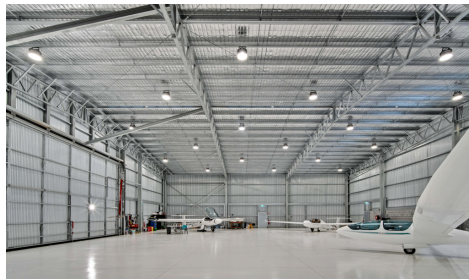
The VALE Aircraft Hangar 000221
